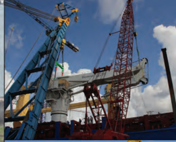
T&T's Derrick Barge "BIG-T" setting legs on a Mobile Offshore Drilling Unit
