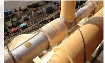
Cargo Pipe Insulation Renewal
