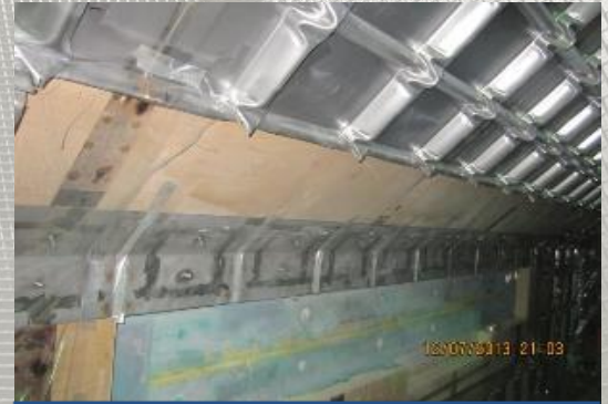
Secondary Barrier Repair
