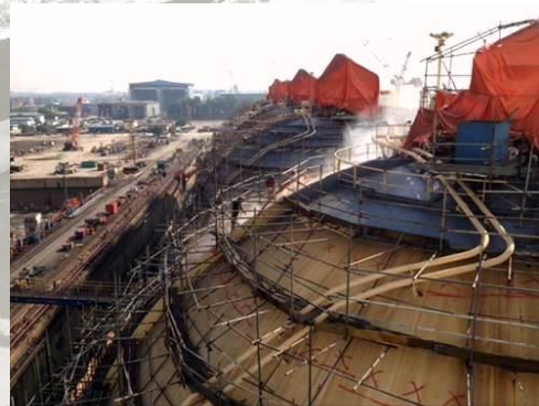
Full dome's staging & dome cosmetic work
