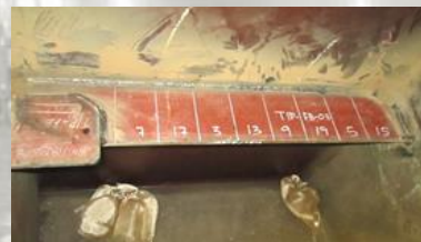
Fit and Weld Process
