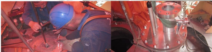
Cargo Tank Radar Gauging System Upgrading
