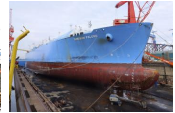
Type of works : Intermediate Survey and BWTS Installation Year : November 2021
