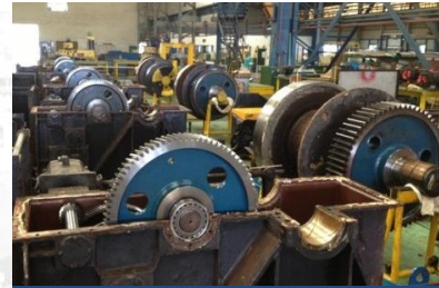
Mooring Winch Overhauling
