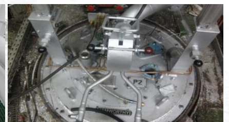
New Boiler Burner System Installation
