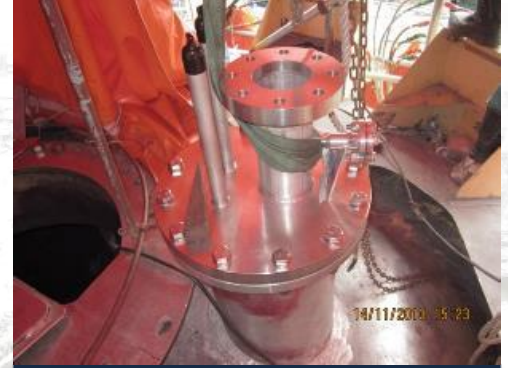
New CTMS / Penetration Installation
