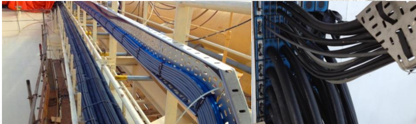
Power & Instrument Cable Renewal
