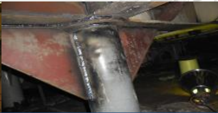
Fabrication Mooring Fairlead Foundation
