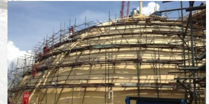
Full dome's staging work
