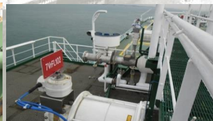
Installation of New Offloading Platform
