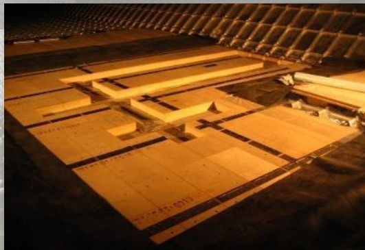
Secondary Barrier Repair
