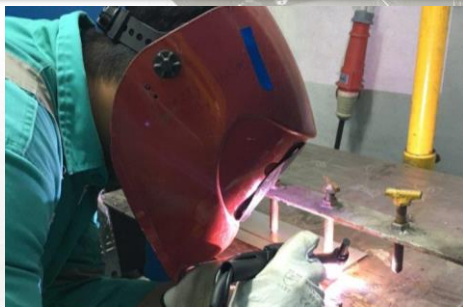
Invar welding training for welder
