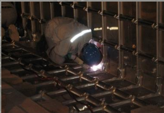
Mark III Membrane Welding
