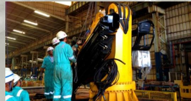
Installation of New Manifold Crane
