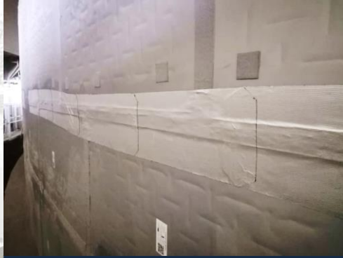
Insulation Repair
