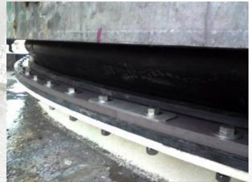
Cargo dome seal renewal
