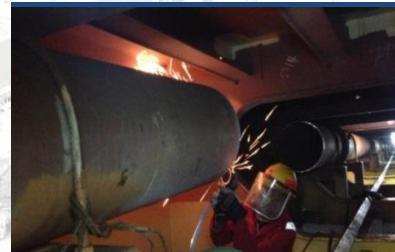
Ballast Line Renewal
