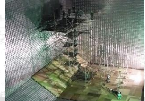
Scaffolding for LNG Cargo Tank
