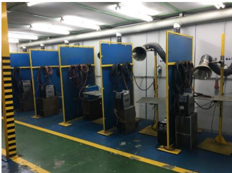
95 m 2 area with 10 welder stations
