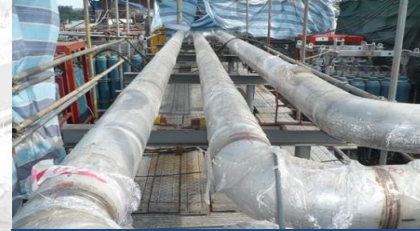
Installation of New Cargo Line
