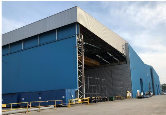
New Centralized Warehouse
