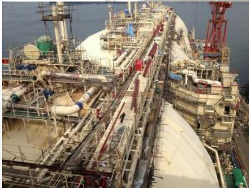
Various Outfitting Works
