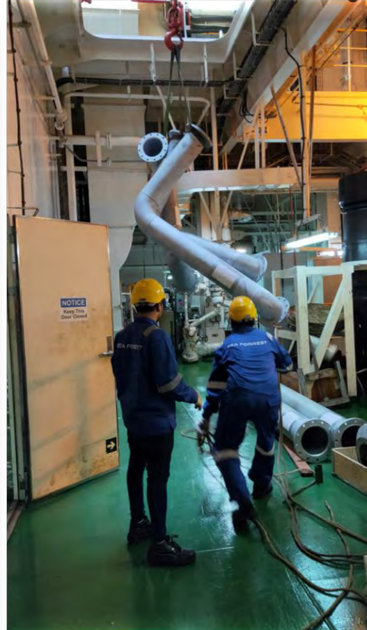
BWT System Vent Pipe Installation Vessel on Voyage from Papua New Guinea to China
