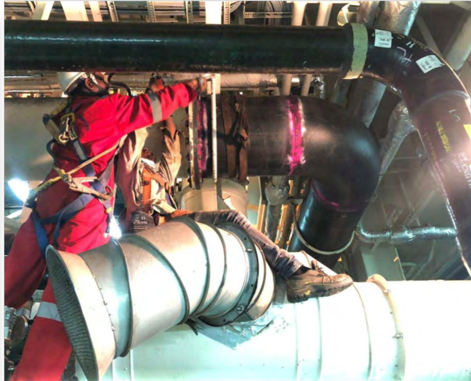
Engine Room Sewage Water Pipe Renewal Vessel at Singapore Anchorage
